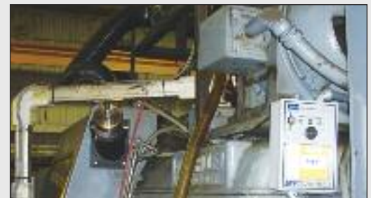
Stat-X automatic generators protecting CNC machine with an externally mounted aerosol unit.
